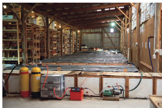
Fig. 3 Part of the basin unit (Photograph: A. Rettel).
